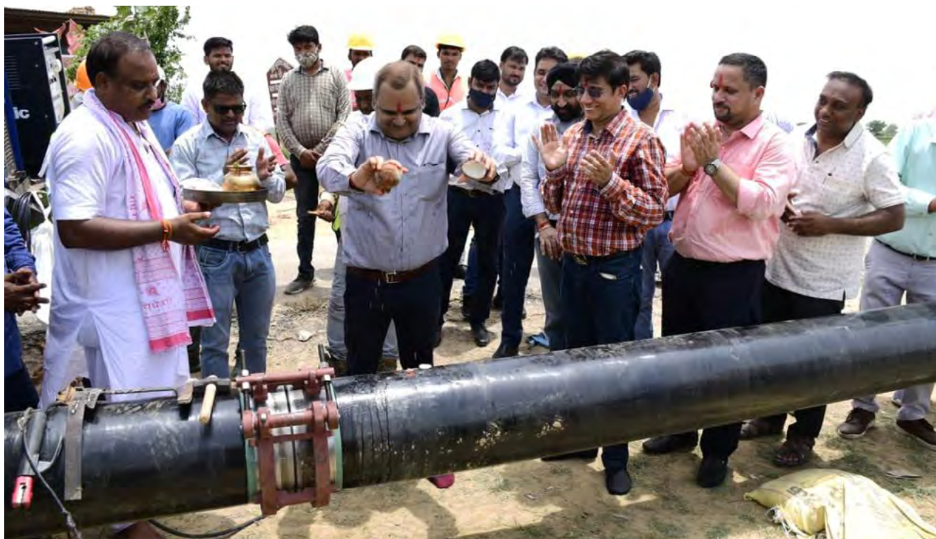
Inauguration of steel pipeline laying work at Hamirpur in Uttar Pradesh.
